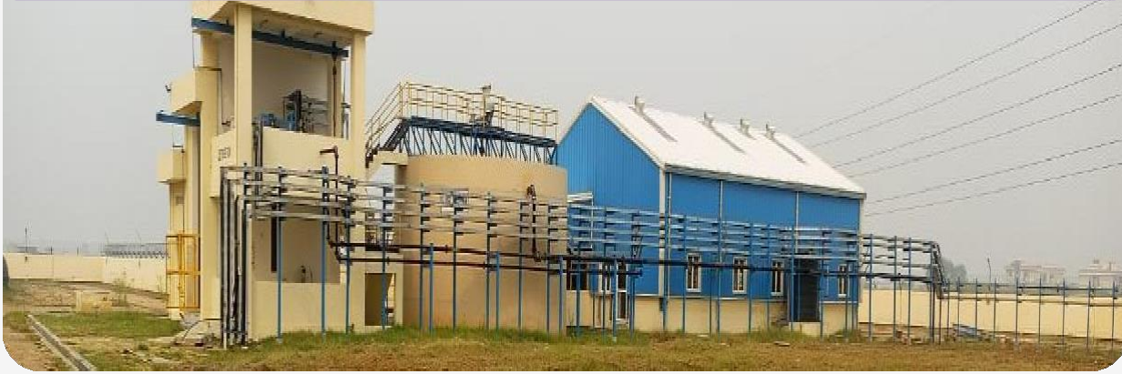
Water treatment unit
