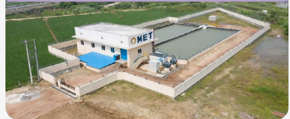
Water Pumping Station
